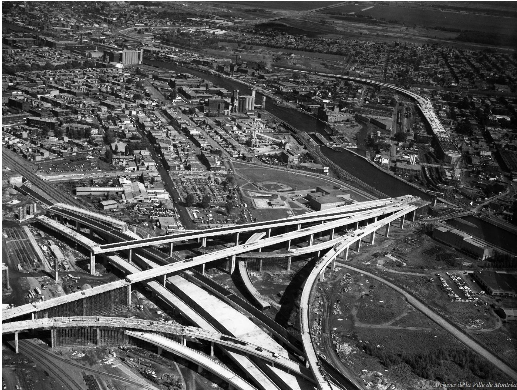
Construction of the Turcot Interchange in Montréal in 1966.
